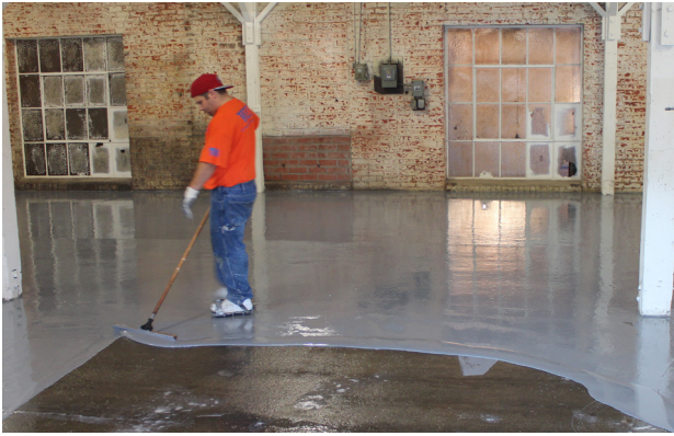
Application of Retro-Coat to a 20 mil total thickness
