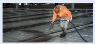
**Example of Nitrile-Modified Asphalt Seams** MonoShield applications utilize a spray-applied nitrile-modified asphalt to seal seams and penetrations, eliminating bottlenecks in performance and installation time.
