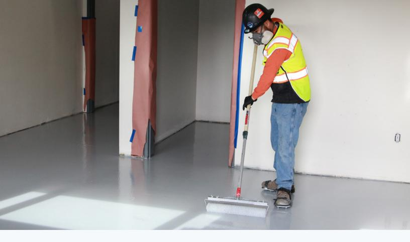
The Retro-Coat® Vapor Intrusion Coating System is a chemically resistant coating technology which protects existing structures from the threat of contaminant vapor intrusion. Retro-Coat is installed on top of existing concrete and provides a durable, finished surface eliminating the need for additional concrete protection.
