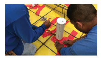
Traditional vapor barrier installations require taped seams which contributes to long construction times and sub-optimal performance.
